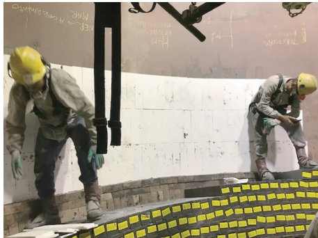
Fig. 2 Installation of the thermal insulation in the Cylinder of BOF#4.
